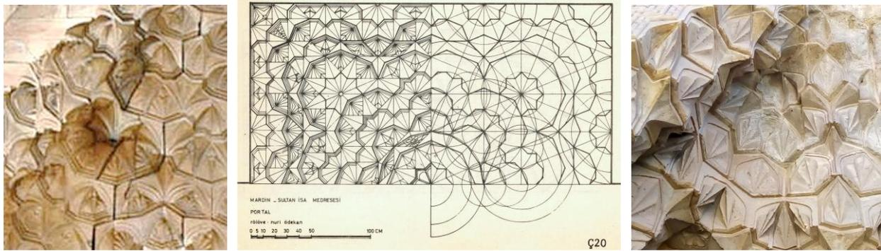
**Figure 5:** (left) Mardin Sultan Isa: the “owls eye” has a small stalactite, (middle) Floorplan Ödekan, (right) Kayseri Sultan Han: the “owls eye” is a small dome-shaped niche.
