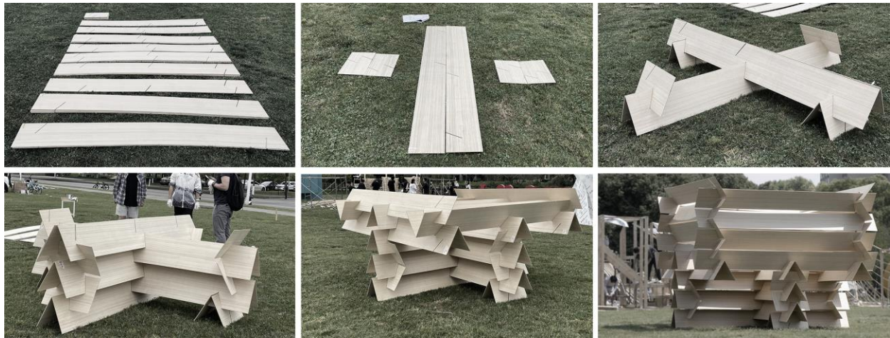
Figure 8: Assembly process of the Half Pavilion.
