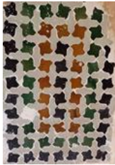
Figure 12: Side arches in Torre de las Infantas tiling
