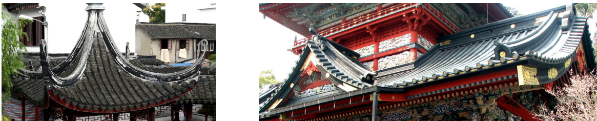
Figure 3 : Roofs at temple complexes in China (left) and Japan (right).
