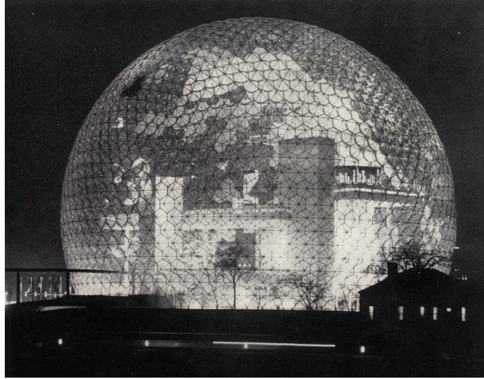
Figure 1: Photograph by Michel Proulx of Buckminster Fuller's Dome at the Montreal Expo in 1967 published in the magazine "Graphis" issue 132 clearly showing the basic hexagonal strut pattern. The more complex interlinking of the double skin structure is also observable but less obviously. It might be of interest to note that only the top hemisphere is actually geodesic. When I returned to Montreal after the discovery of C_{60} with a serious intrinsic interest in the structure, what I wanted to do was enter the cage through a pentagonal opening if possible. To my consternation I could not find one near ground level as I expected. I mentioned this to Ed Applewhite a former colleague of Buckminster Fuller and he pointed out that the bottom half was not actually geodesic! If the reader studies the above image carefully one can indeed see that the hexagons in the bottom half are arranged horizontally whereas in the top half they curve along geodesics. I assume that this is so the structure of the struts at ground level is horizontal, so simplifying construction problems.
