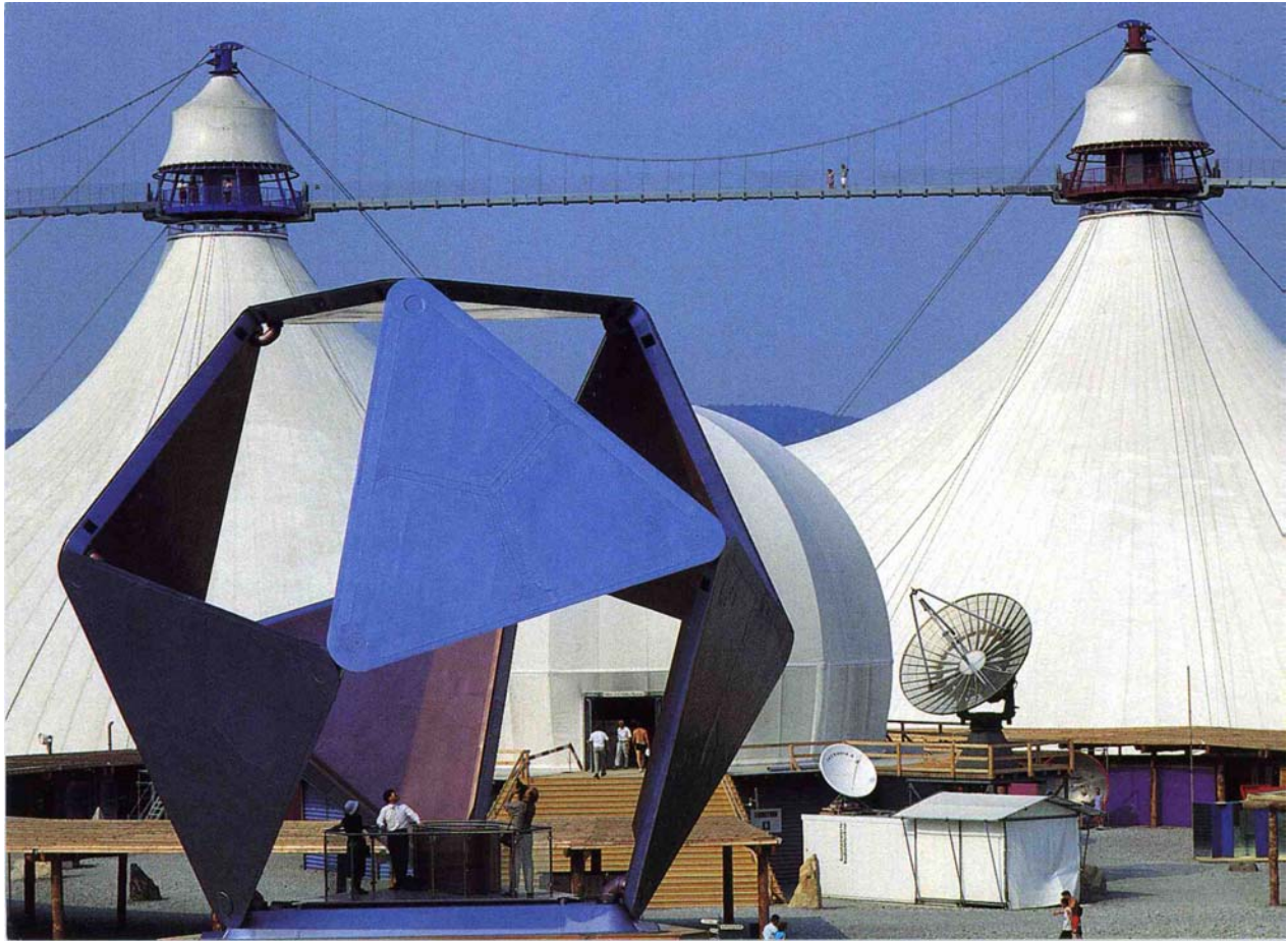
The “heureka” polyhedron. Symbol of the Swiss national science expo 1991. It was a giant “Jitterbug” with a side length of 8 meter (26 feet). Transformed hydraulically from an octahedron to an icosahedron into a cuboctahedron [5]
