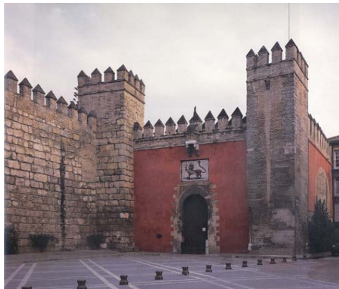
Figure 0. View of the Lion's Gate in the wall surrounding the Real Alcázar
