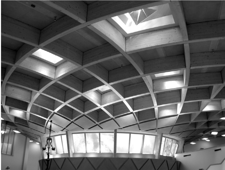
Figure 7 The inside roof structure of The Core
