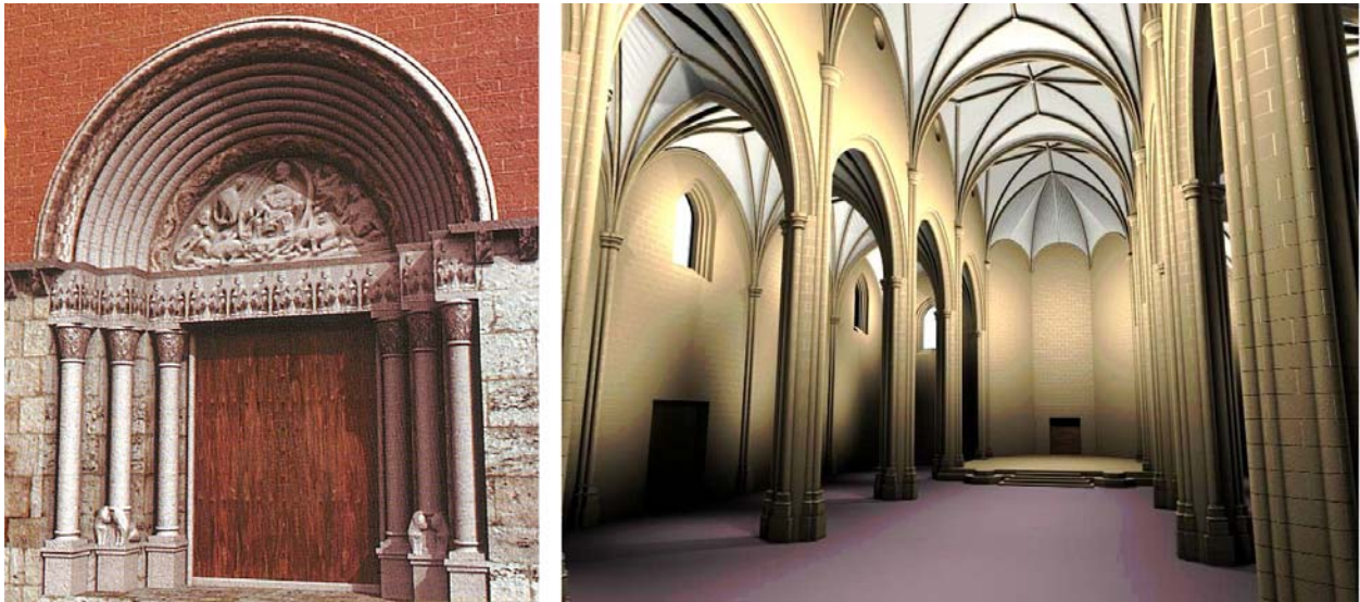
Figure 2: Photogrammetry and topography are two techniques used to take precise coordinates from existing conditions. Photogrammetry is based on the measurement of an object in two photographs taken from separated points towards the same focus. Topography is based on the geometry of an object that looks smaller the further away it is. A Romanesque style portico (left) rendered by means of photogrammetry and the nave of a gothic church (right) measured using topography. Photogrammetry is a technique usually used for detailed, ornamented, models while topography is generally used for larger, less detailed, structures.
