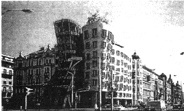
The corner of the National –Nederlanden Building
